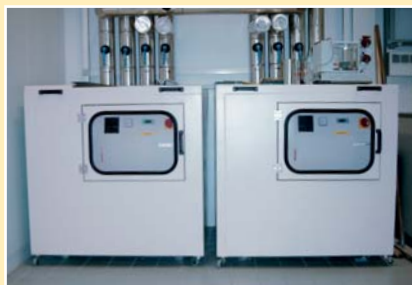
Cooling of several rotary evaporators - sound-proofed, directly in the laboratory
