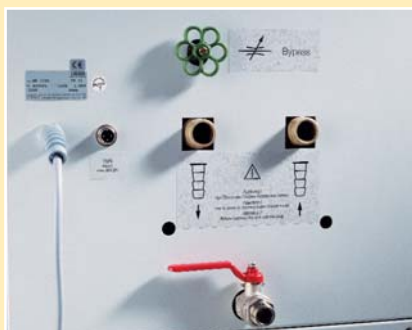
Pump connections with bypass function
